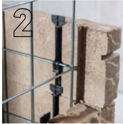
Use connector to attach Tandem Veneers to grid
