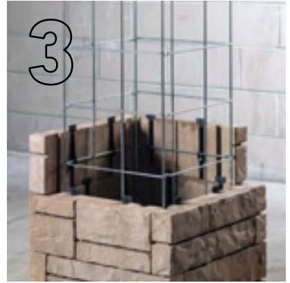
Repeat step 2 and fill with \frac{3}{4} " crushed rock until column is complete
