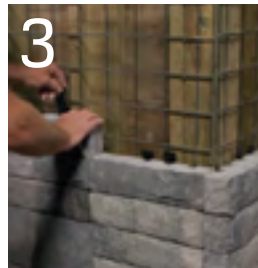
3 Attach Tandem Veneer with Connector
